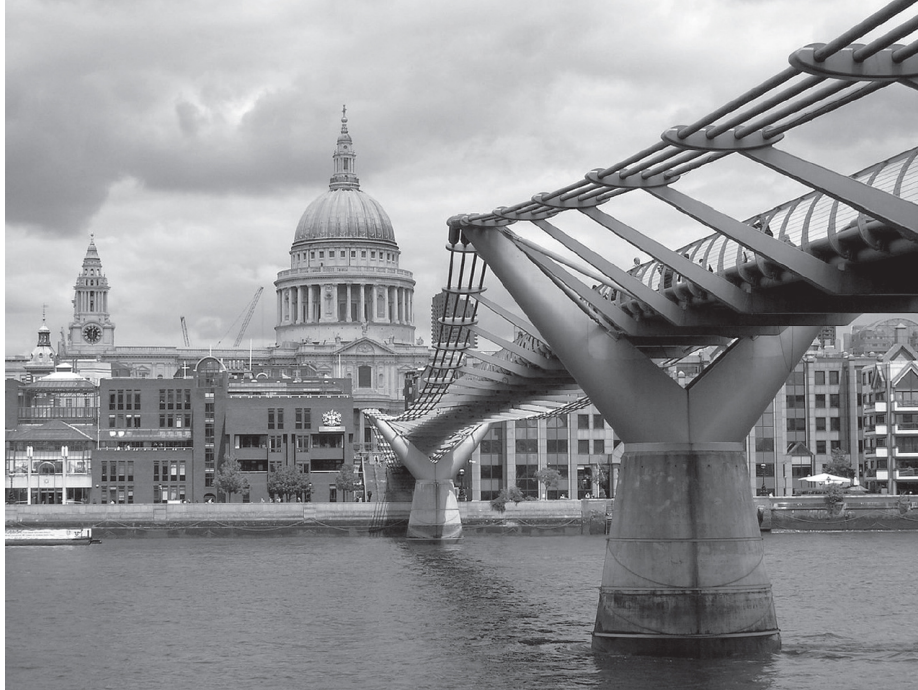
The Millennium Bridge.
