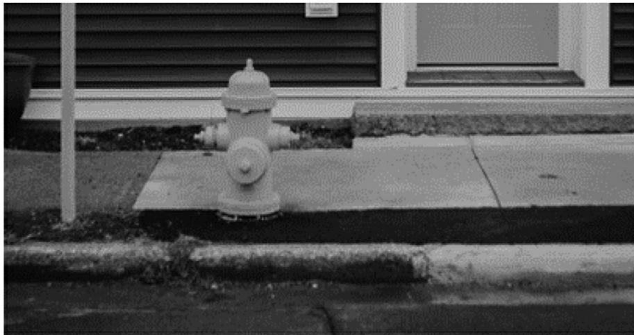
Newly painted hydrant on Little River Road, Flamborough. The project has taken two years to complete
