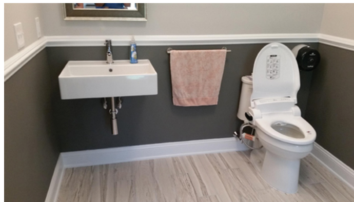
Figure 21-5 Bidet toilet seat and suspended sink. (Reprinted with permission from Gregg Frank.)
