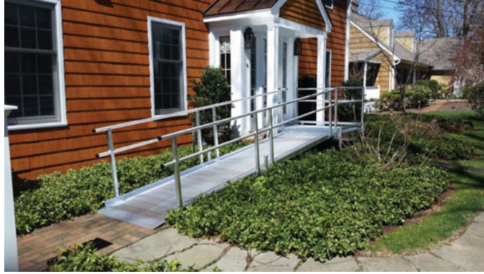
Figure 21-1 Portable ramp. (Reprinted with permission from Gregg Frank.)
