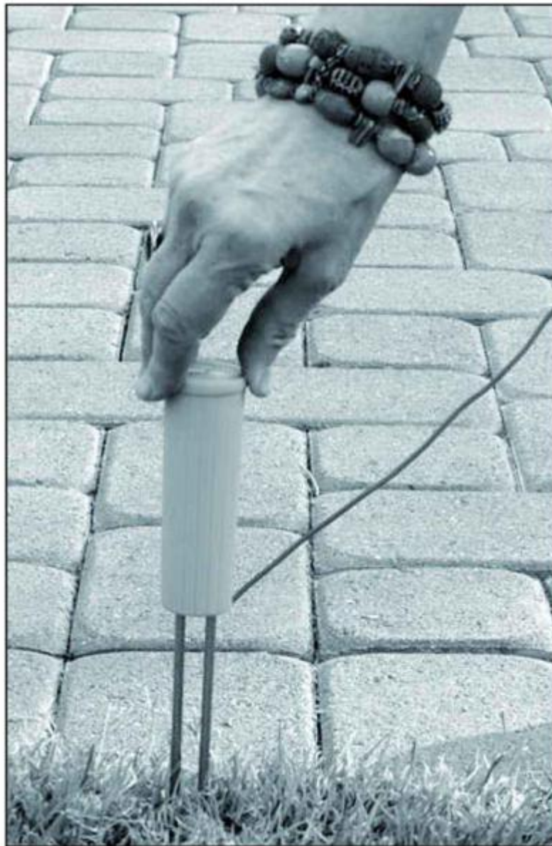
Figure A-1. Placing ground rod in Earth.
