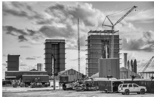
The construction tents and high bays in Boca Chica
